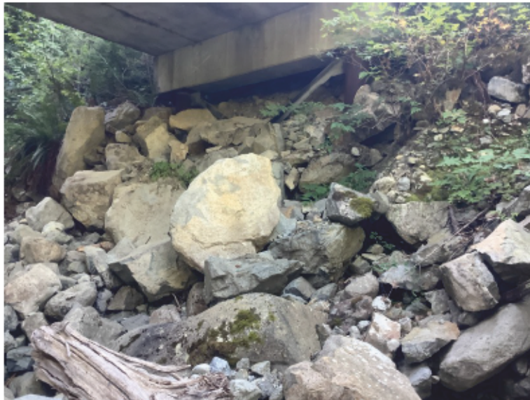
Left Bank Abutment when facing downstream
