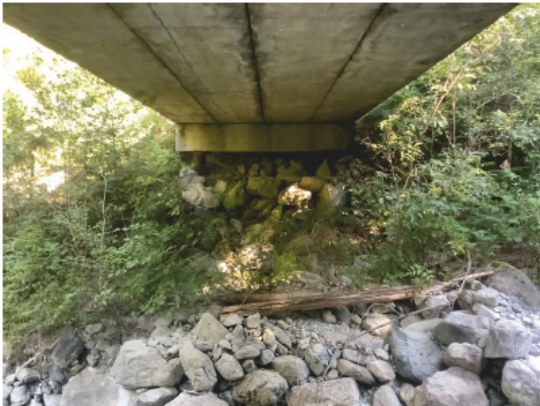
Right Bank Abutment when facing downstream
