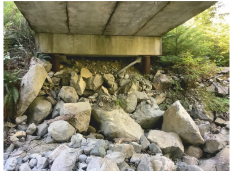
Left Bank Abutment when facing downstream
